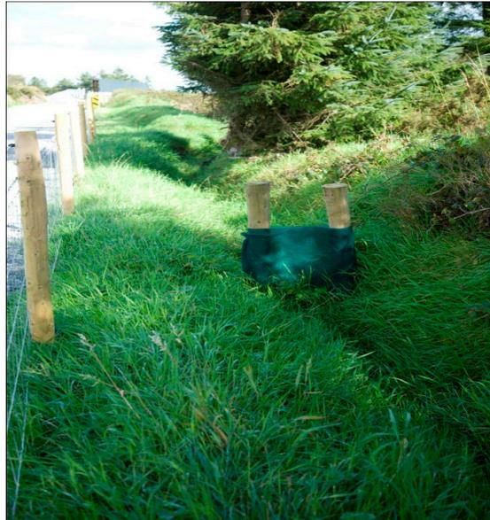
**Figure 3-5:** Silt trap across grassed swale
