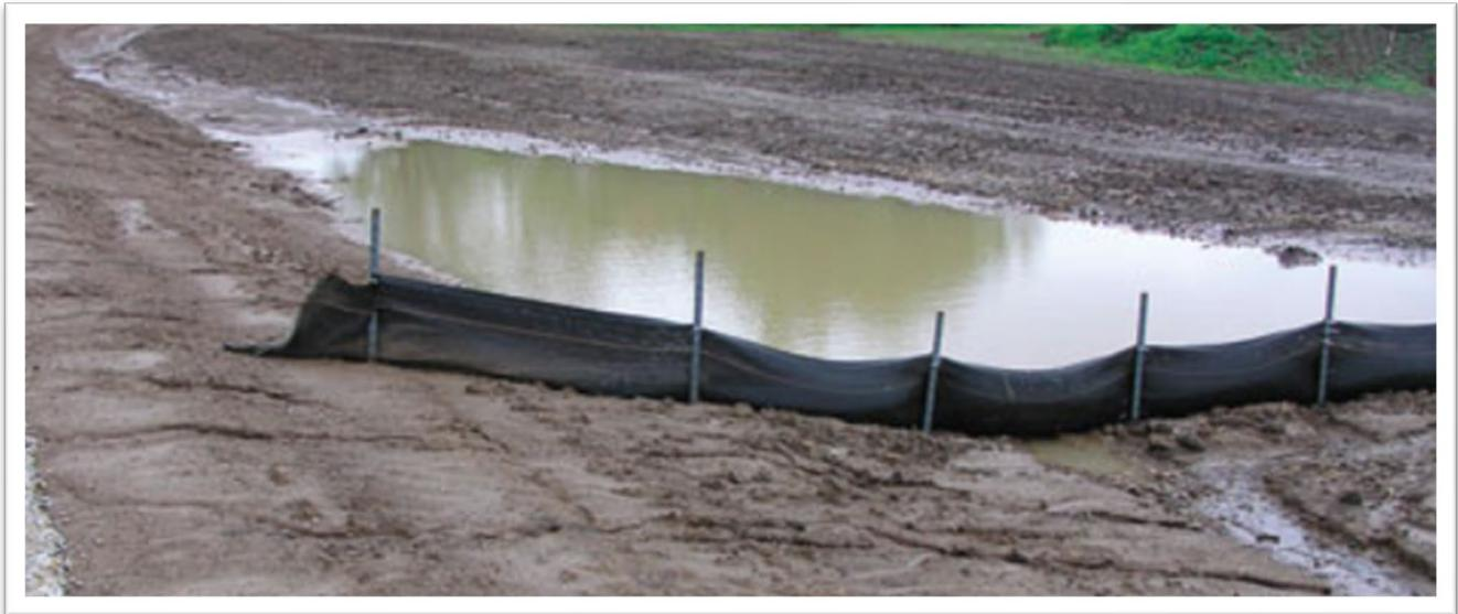
**Figure 3-7: Silt Fence**
