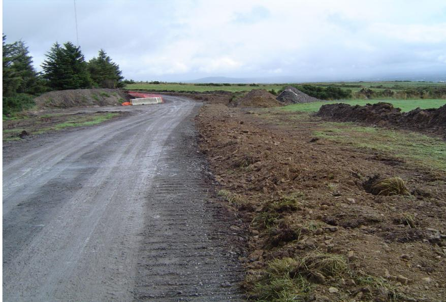
**Figure 3-8: Backfill over cable trench**
