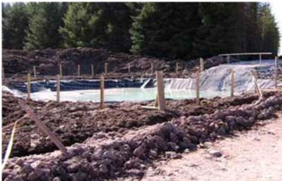
**Figure 3-9: Lined Settlement Lagoon for Concrete Washout Facility**
